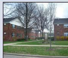
GLEN ELLYN Iron Gate Apartments 180 Units
