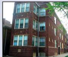
ALBANY PARK 3105-3109 W. Argyle 9 Units
